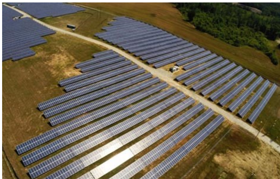
FLS Solar's Fairmont facility in North Carolina | FLS Solar
