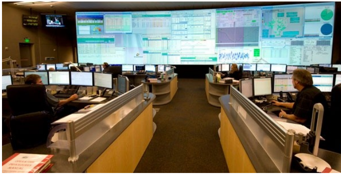
ERCOT control room | ERCOT
